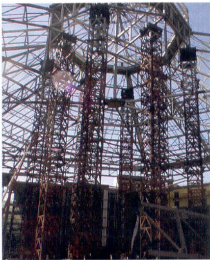
FabArc Steel Supply Inc. has grown to include two manufacturing plants with a total fabricating and inventory area of more than 700,000 sq. ft.
