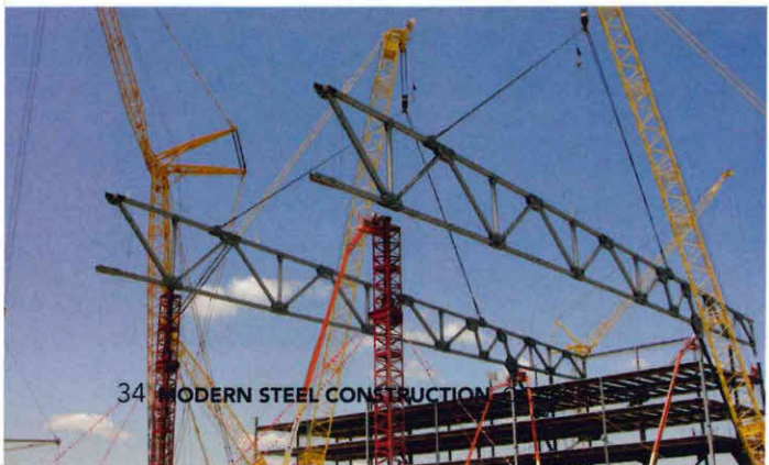
◀ With the first truss section in place but still supported by the crane, the second truss section was hoisted into place.
